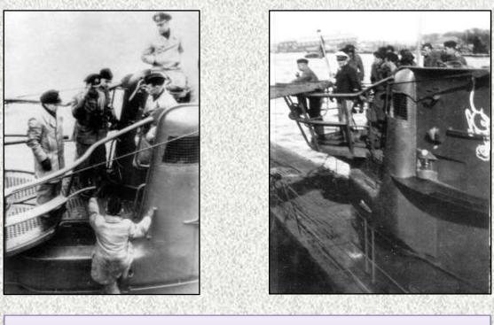
Above left (26): The large air trunk on the starboard side (another was present on the port side) and the grill are apparent in this  $3^{rd}$  November 1940 image of U 47. The pattern of the square drainage holes on the floor of the tower are also noteworthy since they cannot usually be seen in most photos.
