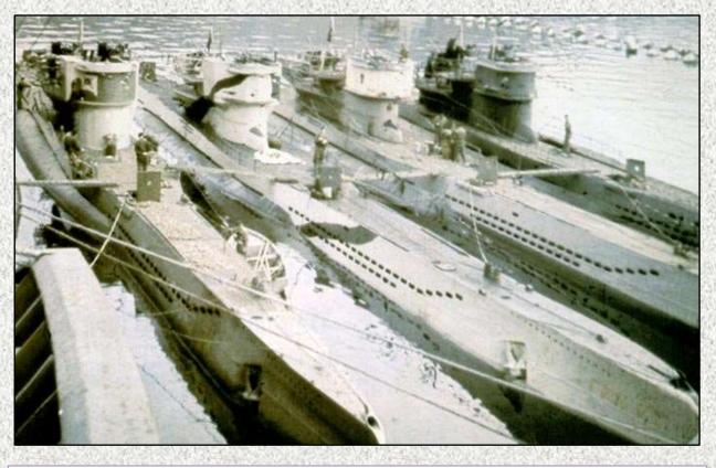
Above (10): In this extremely useful colour image, taken in Hammerfest on the 30<sup>th</sup> July 1944, each of the four boats has a different configuration. This presents a perfect illustration of the lack of standardisation in the late war period. The only boat in this photo which has the same arrangements as Revell's RV5045 kit is U 997.
