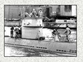
Above (D5): On the IICs there were 19 vents to the rear of the two dots. On a number of IIDs there were 18 vents, which is a useful point of differentiation. On U 149 and U 152 there were 17 to the rear of the two dots.
