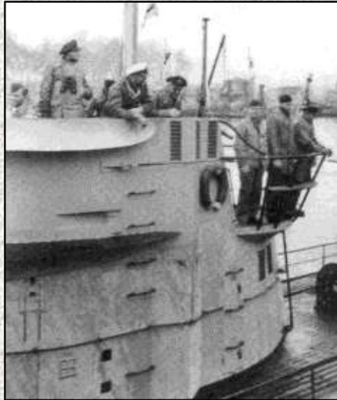
Above (6): The port side of U 108 in December 1941, showing how style Y was separated into three sections due to the curved periscope rod aerial fairing. Note the feature towards the bottom left of this image; this includes a door with a square marker plus two square vents to allow water to drain in and out. This feature was present in some IXBs and all IXCs.
