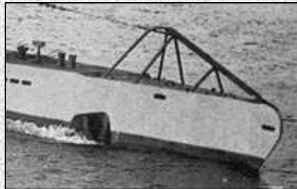
Above left (45): The straight edge of the net cutter can be seen on the boat on the right, which is the IXA U 38.
