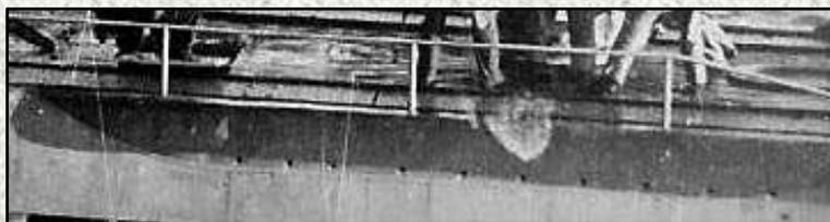
Above (50): The hull breakwater on an IXB showing ten small round drainage holes. The third hole is not equidistant between the second and fourth hole and is slightly elevated above the rest. U 123 did have the ten holes but they were all equidistant. These holes were normally retained when the hull breakwaters were removed.
