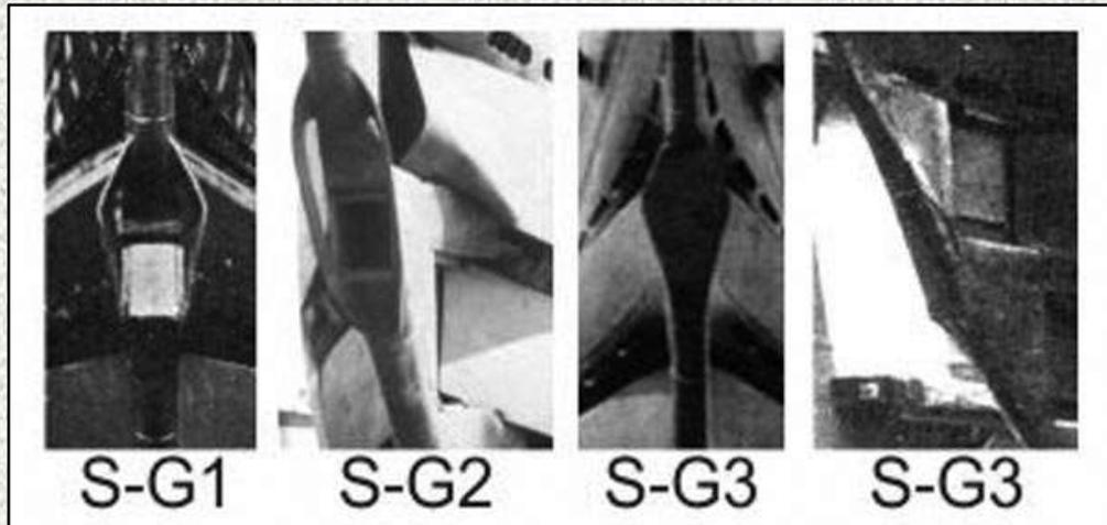
Above (35a-35d): The three styles of S-Gerät on the stem of early to mid-war IXCs. There are two views of S-G3. The frontal view of S-G3 is U 158 and the side view is of U 194.
