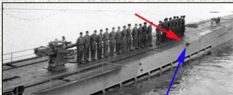
Above (40): U 106 in position 2, with the blue and red arrows showing very little separation between the fairlead and bollards.
