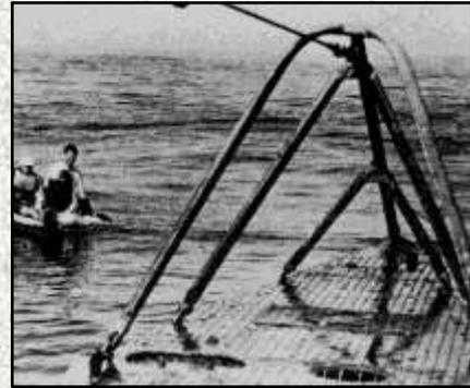
Above left (43): The upper net cutter on this wartime shot of the Type IXA U 37 has ten serrated edges rather than the nine edges on Revell's early war IXC kit.
