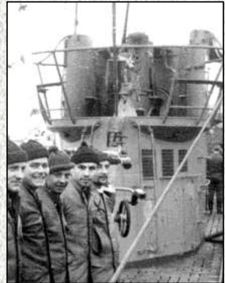
Above (28): This later shot of U 108 shows that the metal seats have been replaced by a ledge low down on the bulwarks and on each side of the periscope housing.
