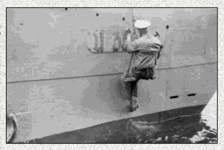
Above (33): In mid August 1939, a crewman removes a pre-war identification bow plate from the VIIA U 35 in readiness for the commencement of hostilities. At the bottom left can be seen the two-digit welded numbers, directly in front of the anchor recess, without white paint. Welded numbers have also been seen on U 30 and U 31 so it is likely that all ten VIIAs had this feature.
