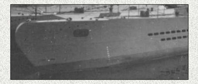
Above (7): Another image taken in the pre-war period, this time of the original VII (VIIA) U 35. The white numbers are clearly shown against the medium grey upper hull paint. Some of the numbers are not so clear against the dark grey lower hull paint. The numbers would have been present but may be obscured beneath a scumline or any slime that tended to accumulate just below the waterline of boats sitting in harbour. On VIIAs, the numbers on the bow ran down to the top of the lower torpedo door.
